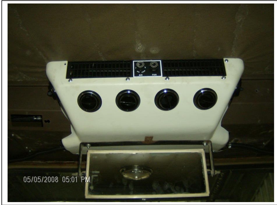
New evaporator mounted on ceiling
